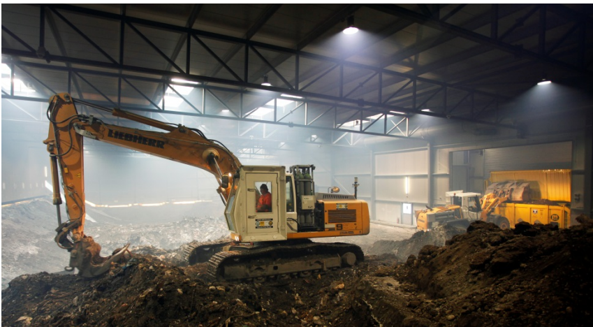
Deponie Pont-Rouge, Aushubhalle (Foto: CIMO)
